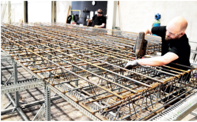
Double wall assembly on the Skew Jig System
